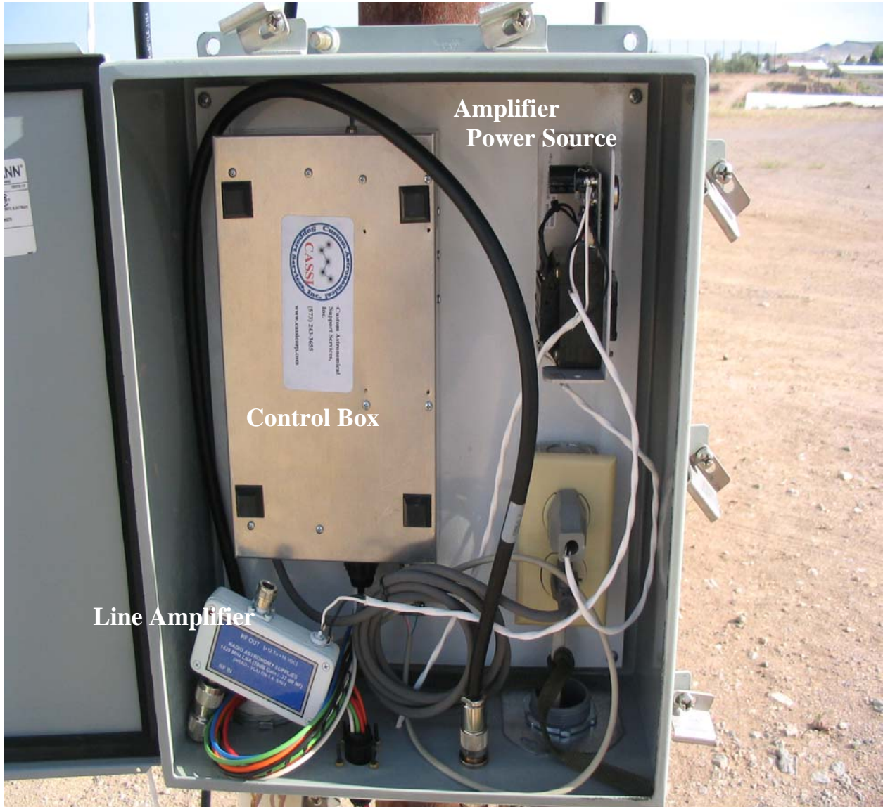
Fig. 7.— Inside the weather proof boxes attached to the telescope bases.
