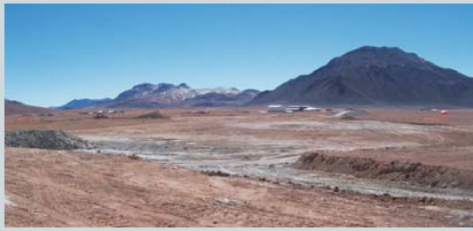
Figure 3. Antenna station excavation has begun at the center of the array at the 16,400-foot level. The Array Operations Building is in the background; the newly completed transporter shelter is to its left.
