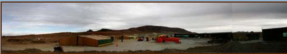
Figure 2: A panorama of construction at the Atacama Compact Array (ACA) site. Concrete poured for foundations must be cured at a controlled temperature inside tented structures (center). The ACA has 22 foundations and will be used for initial astronomical validation.
