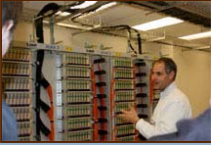
Figure 3: Backend lead Fabio Biancat Marchet shows the newly completed fiber optic patch panel in the AOS Technical Building to members of the AAER panel.
