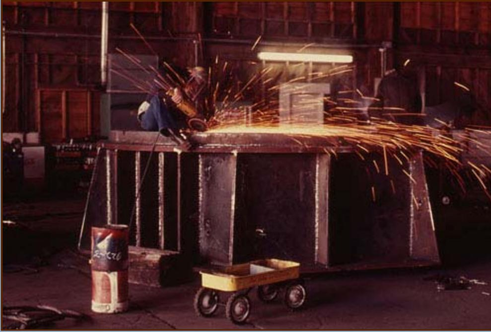
Machining the azimuth bearing box for Very Large Array (VLA) antenna #4 in Hobbs, NM, January 1976. The VLA antenna contractor was E-Systems, Garland Division, Dallas, Texas. They used a fabrication plant in Hobbs belonging to Structures, Inc. to fabricate the various steel antenna structural parts, and parts were then shipped to the VLA for final assembly. Thanks to Lew Serna for background information on this photo.
