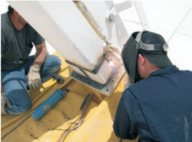
Figure 1. Patching a subreflector support leg on the VLBA antenna at St. Croix.
