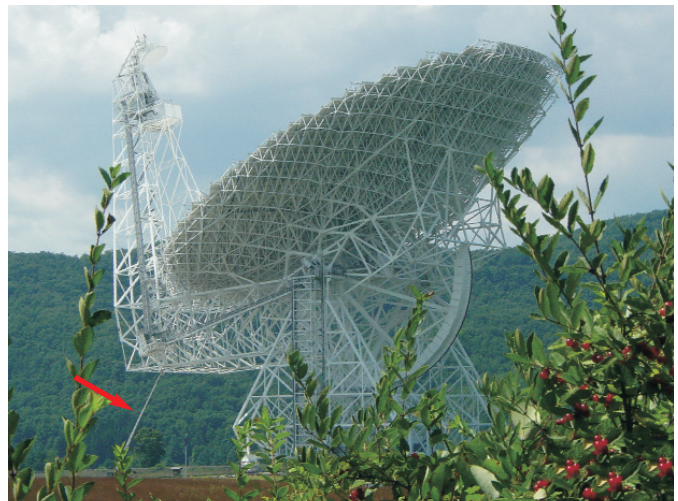
A summer painter works from a manlift over 100 feet from the ground to reach the bottom of the feed arm of the GBT (red arrow indicates the lift).
