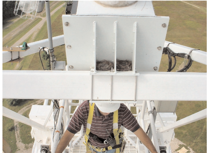
Industrious birds built these nests on top of the GBT. While this photo shows them sitting vertically, this perch tips nearly horizontal during observing! Operations Division Head Bob Anderson is visible just below the nests.
