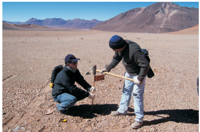
Figure 3. During August, each of the new antenna stations in the newly designed inner configuration was staked by an on-site team. Problems were reported back to Conway, who then implemented small changes to perfect array performance. Here, station 136 is staked.
