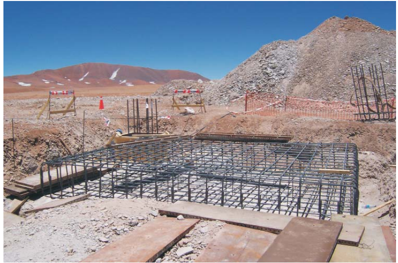
Figure 1. Construction on the Technical Building at the Array Operations Site. This building will house the ALMA correlator, local oscillators, and all local hardware.
