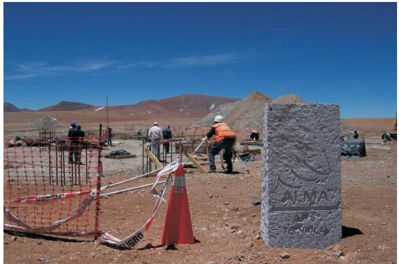
Figure 2. Construction site with the ALMA corner stone in the foreground.
