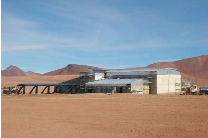
Figure 1. The Array Operations Site (AOS) Technical Building (TB) exterior, which will house array electronics such as the ALMA Correlator, has been completed. It is one of the highest-altitude (16,570 feet), highest-technology buildings in the world.
