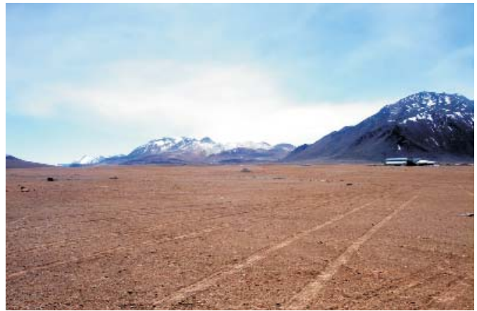
Figure 2. The AOS TB as seen from the future center of the array. As construction progresses, this area will contain the antenna pads for the compact configuration of ALMA.
