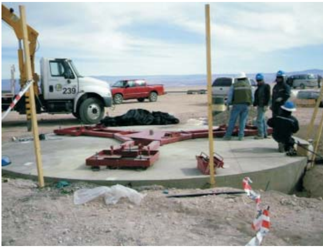
Figure 2. Bottom section of antenna jig installed and bolted to the foundation, and awaiting the first VertexRSI antenna at the OSF site.
