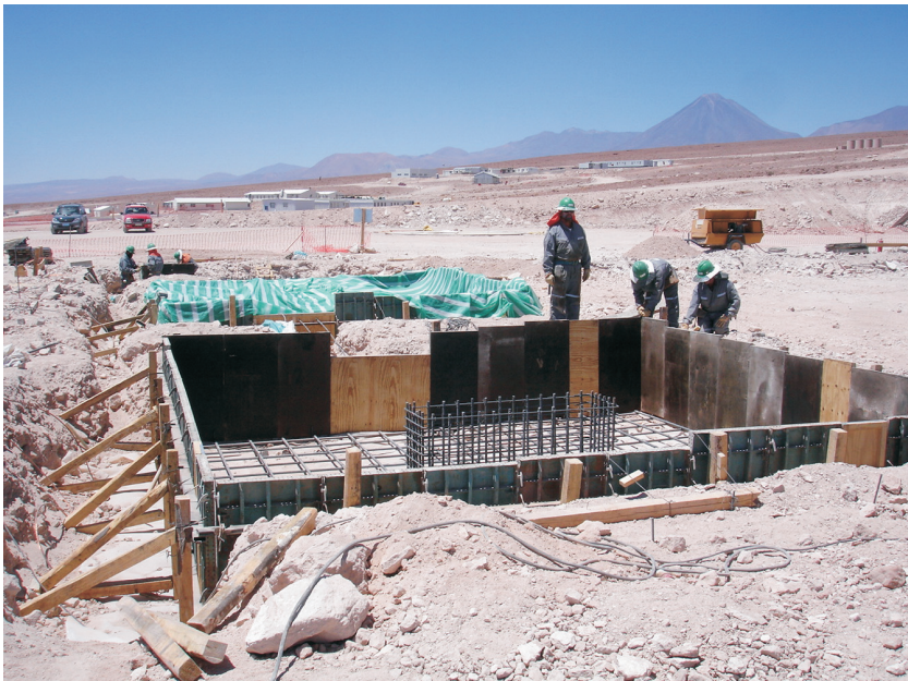
Figure 2. Work on the building for the VertexRSI Site Erection Facility has begun in preparation for receiving the first production antenna in early 2007. The ALMA camp is in the right background, in front of Licancabur.
