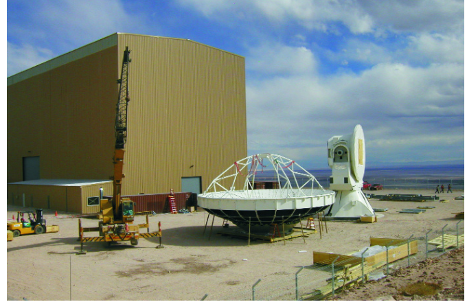
Figure 2. The first ALMA production antenna at the OSF: the VertexRSI pedestal stands on its pad to the right of the partially assembled backup structure, and in front of the VertexRSI site erection facility.
