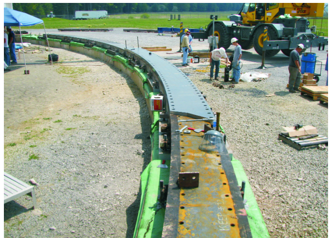
Figure 4. First three base plates and wear plates being placed in position.
