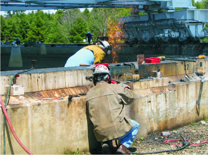
Figure 1. Removal of old welds.
