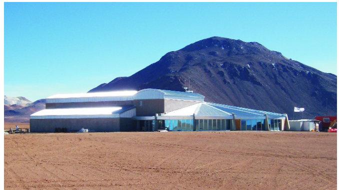
Figure 4. The Technical Building at the Array Operations Site.
