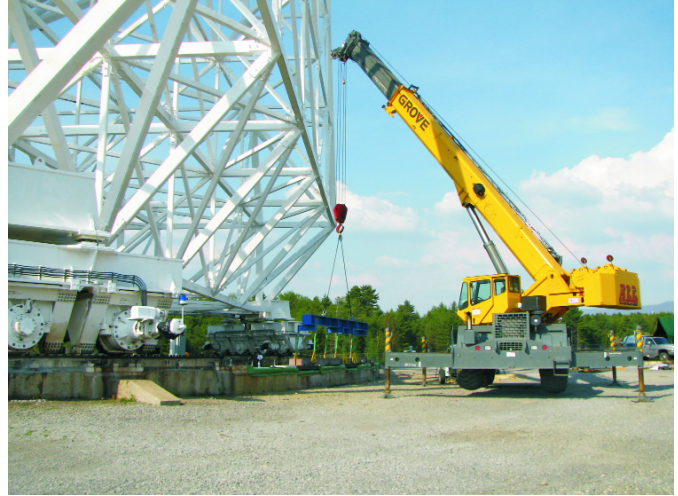
Figure 3. Setting of the first new base plate onto the foundation.
