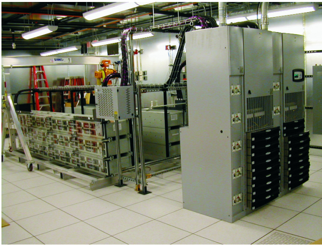
Figure 2. 48 VDC power plant for the WIDAR correlator.
