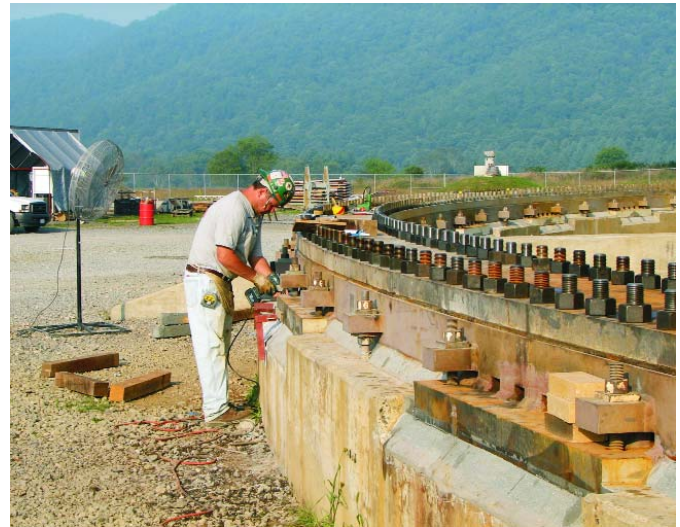
The last sections of track being formed for grouting on August 30.
