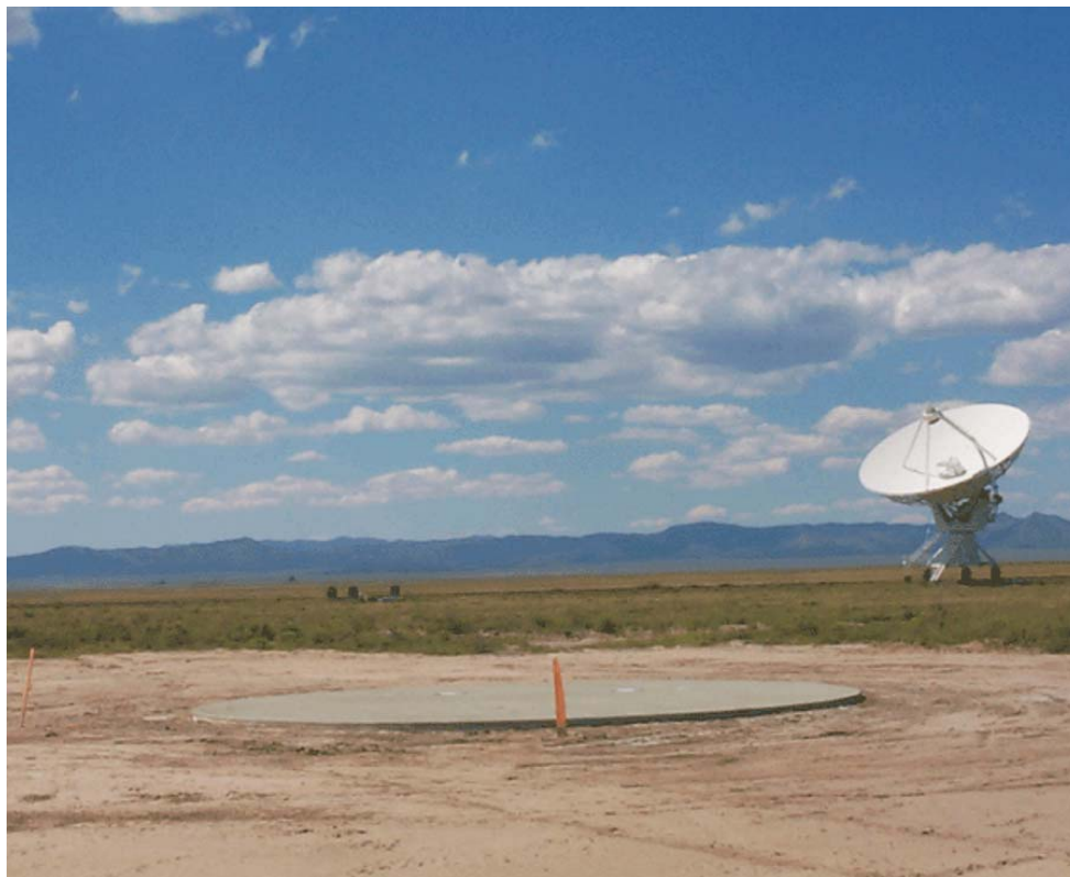
Completed foundation at the VLA site where the VertexRSI antenna components will be erected this spring. Extensive tests are planned to verify that the prototype will meet all of ALMA's requirements.
