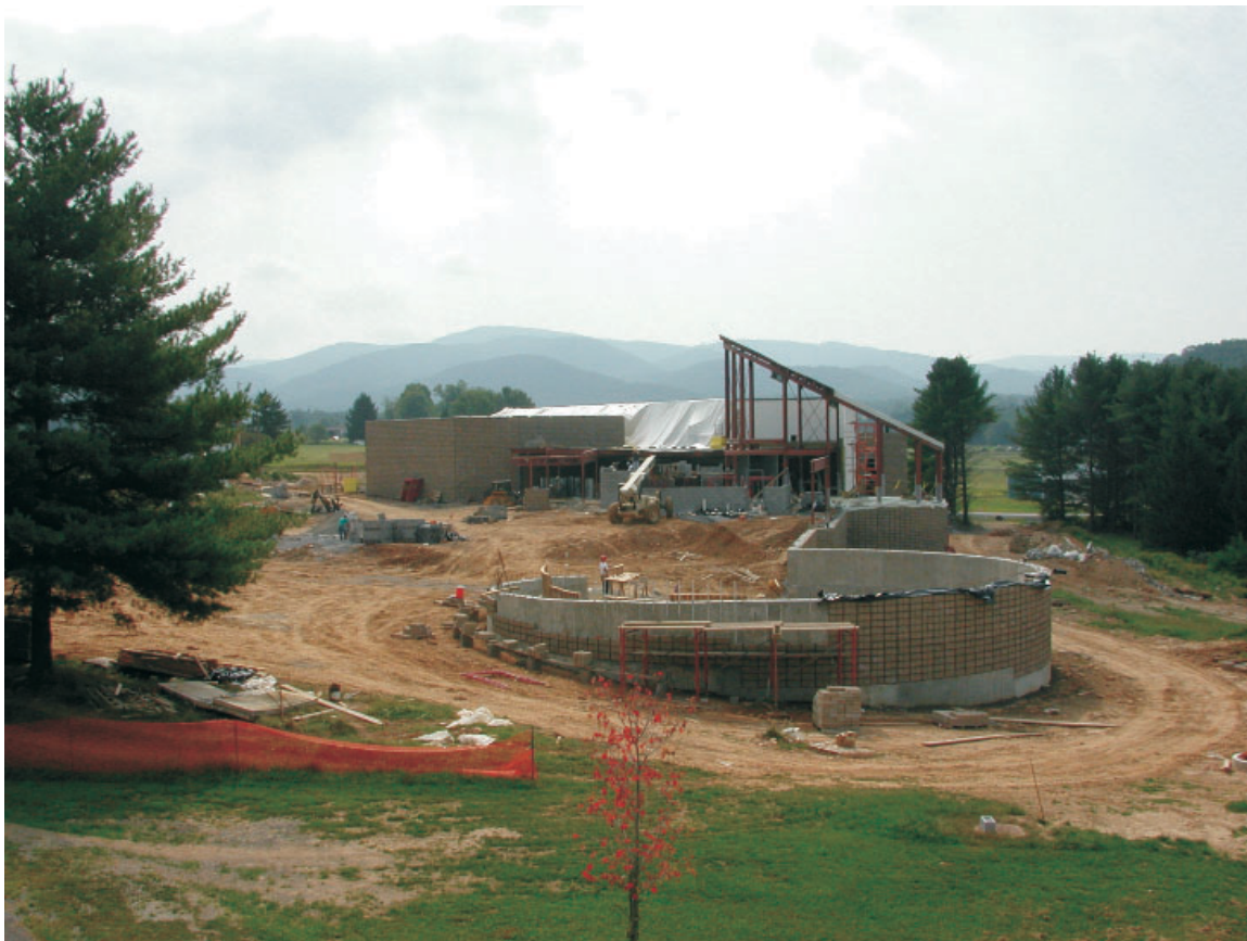
Construction progress of the Green Bank Education and Visitor Center.
