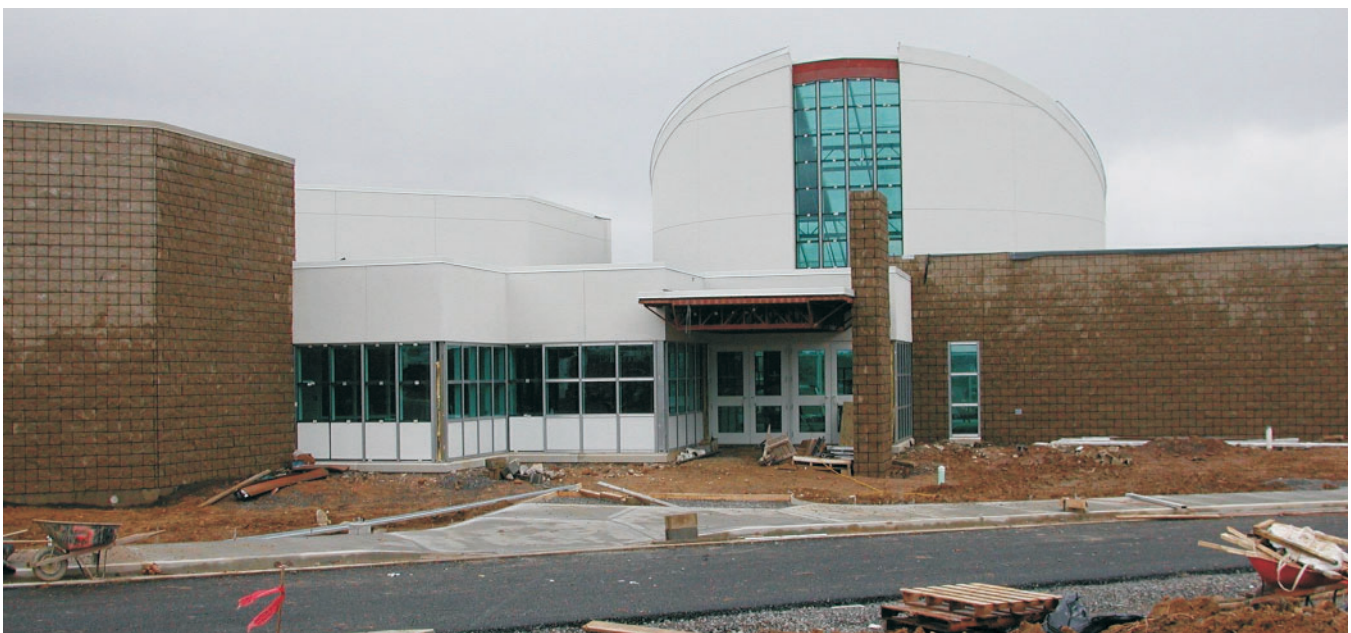
The Astronomy Education and Visitor Center (AEVC) construction is moving along nicely.
