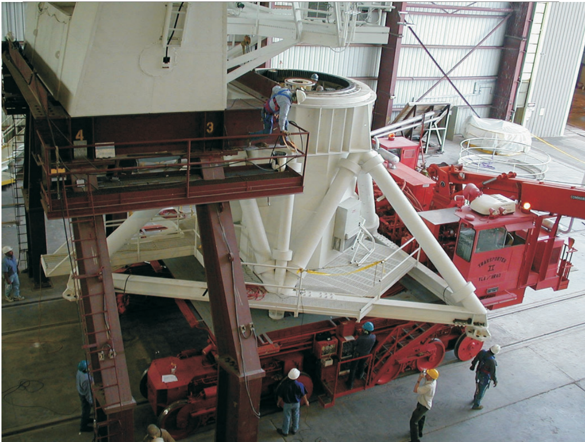
Bearing change on Antenna 7 was successfully replaced during the week of September 16, 2002.
