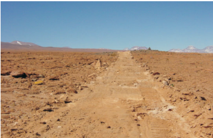
Construction of road from public highway to ALMA site. Photo courtesy of Jorg Eschwey (ESO)
