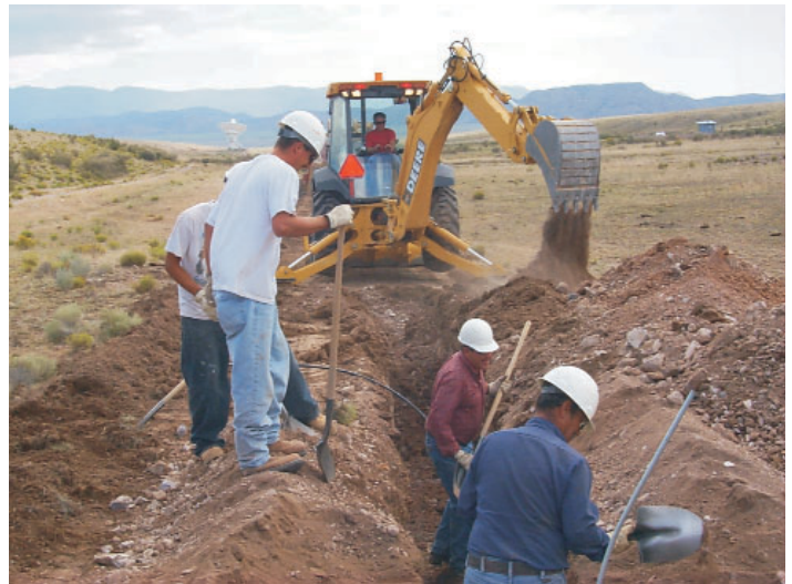
Figure 4. Fiber installation crew working at the end of the east arm. The antenna in the background is on station AE9.
