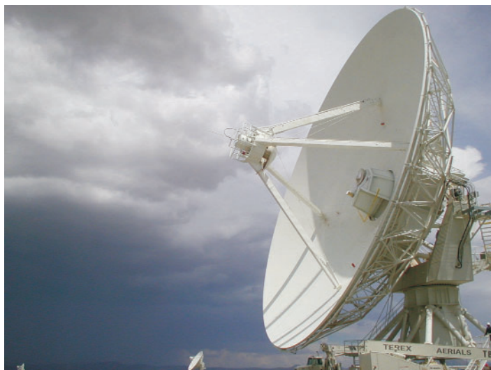
Figure 1 The EVLA Test Antenna on the Master Pad with the new feed cone installed.
