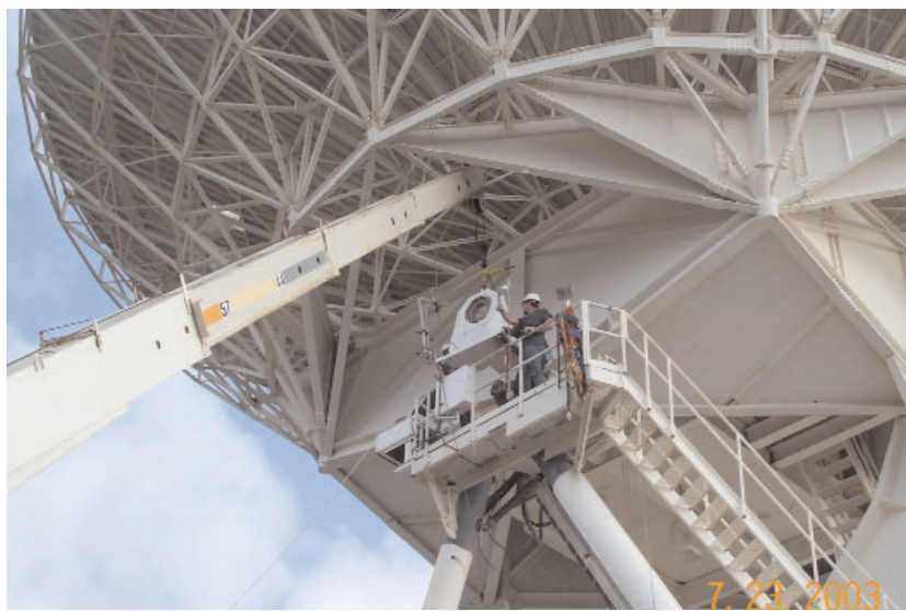
The installation of the new elevation bearing and its pillow block mount at the VLBA antenna in St. Croix. Photograph by Pete Allen.
