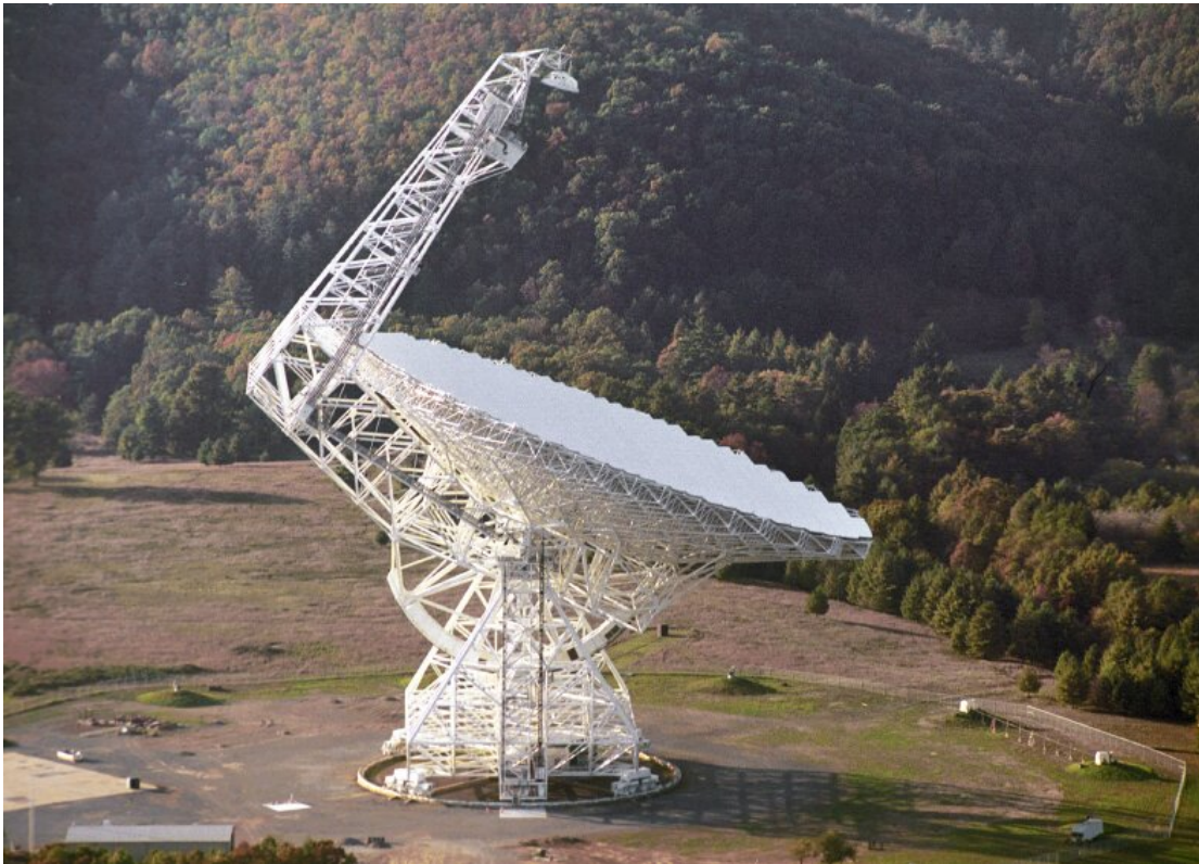
Figure 4.1.1 The Robert C. Byrd Green Bank Telescope has a 100 m diameter unblocked aperture and a computer-controlled active surface.
