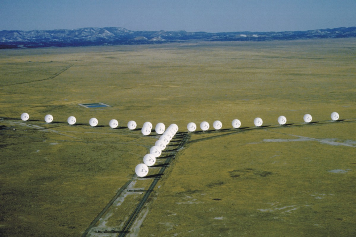
Figure 4.2.1 The smallest VLA configuration spans 1 km on the Plains of San Augustin at 2,100 meters (7,000 ft) elevation.
