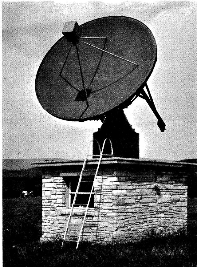
**FIGURE 18.** The 12-foot precision paraboloid that has the same f/d ratio as the reflectors of the 85-foot and 140-foot telescopes.
