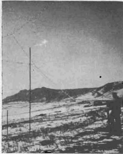
Antenna array for solar-flare detection uses two parallel half-wave folded dipoles, spaced one half-wave apart and driven in phase
