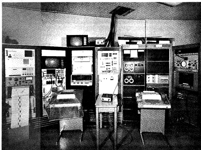
The complex equipment in the Data Room of the 120-inch telescope.
