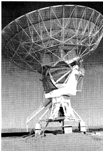
Completed Antenna number 14 on Master Alignment Pad.
