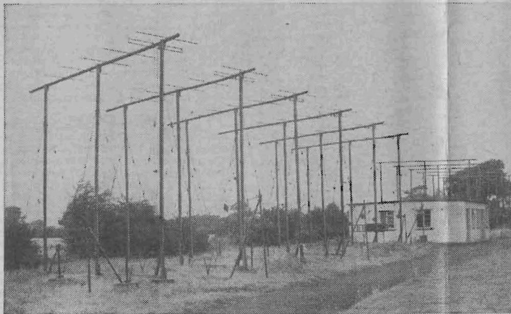
The aerial system used for the continuous survey of meteors by the radio echo technique. In the small building is the apparatus which has now been working for several years and has provided information about meteoric activity uninterrupted by cloud or daylight.
