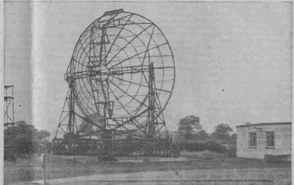
received radio waves on a wavelength of about two metres. This instrument could readily be pointed to different parts of the sky. With it Reber confirmed Jansky's discovery that radio waves were reaching the earth from outer space, and he made the first
