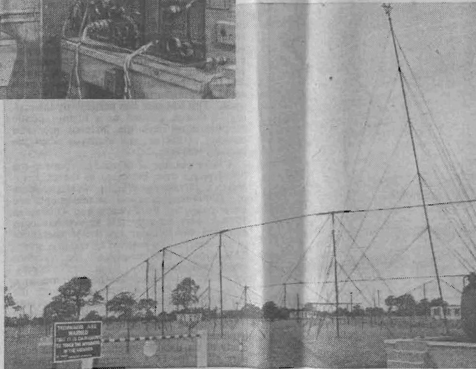
A recent photograph showing part of the 220ft. aperture fixed radio telescope which has a paraboloidal surface formed by a series of wires supported around the perimeter by posts 24ft. high. The aerial at the focus is carried on a 120ft. mast, which is tilted to displace the beam from the zenith. Above: Recording apparatus used with the telescope; the chart shows that the radio star in Cygnus has just passed through the beam of the aerial system.
