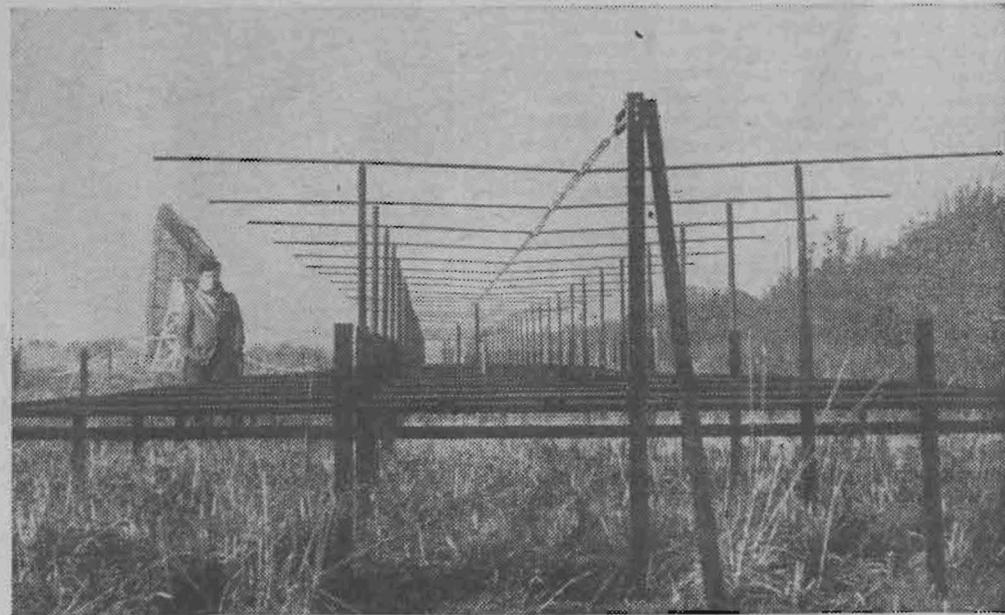
One of the interferometer aerials used by Ryle at Cambridge in the work leading to the discovery of radio stars. Two series of rods—or broadside arrays—separated by several hundred yards on the ground are an alternative to the paraboloidal type of radio telescope.
