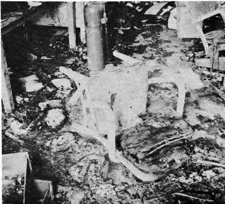
Center of Room 310
