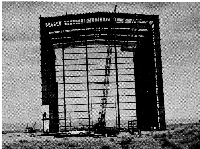
Erecting the Antenna Assembly Building.
