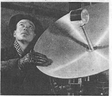
(Photo from Allis-Chalmers Manufacturing Co.) Wilson manipulates directional concave disk antenna in connection with radio apparatus used in receiving impulses from the sun.
