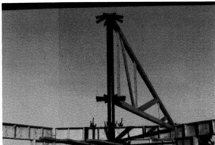
Up goes first roof beam on October 13, 1976.
