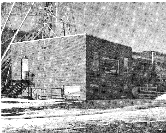
The new addition to the 300-ft control building was completed in December 1971.
