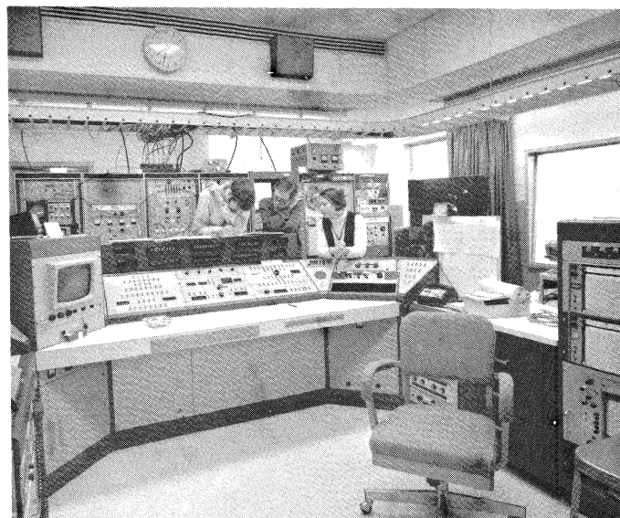
The control center inside the new addition to the control building.
