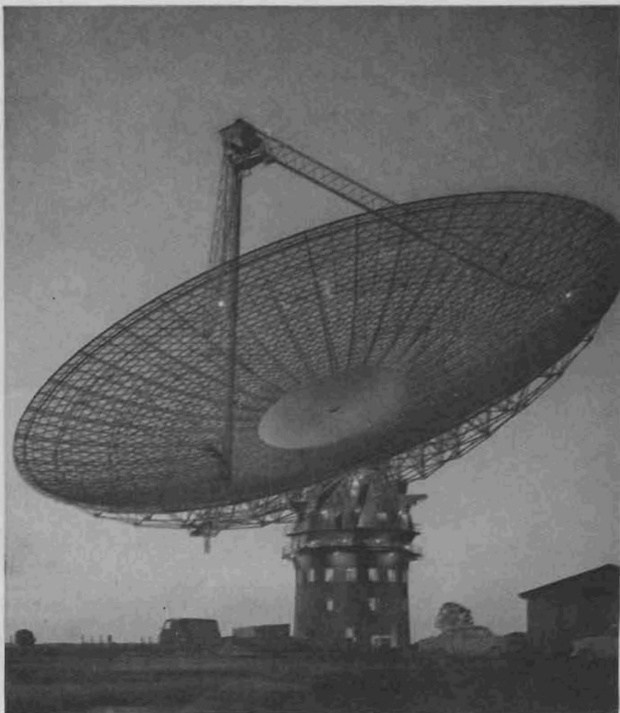
LARGEST SCANNER in Southern Hemisphere is 210-ft. dish at Parkes, New South Wales. Australians are using it to map Earth's own galaxy.
