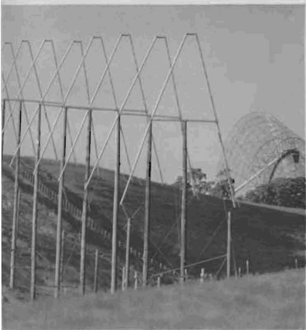
TREE FARM of 40-ft. booms at Stanford receives radar impulses bounced off moon by transmitter. The dish ( right ) is for higher frequencies.
