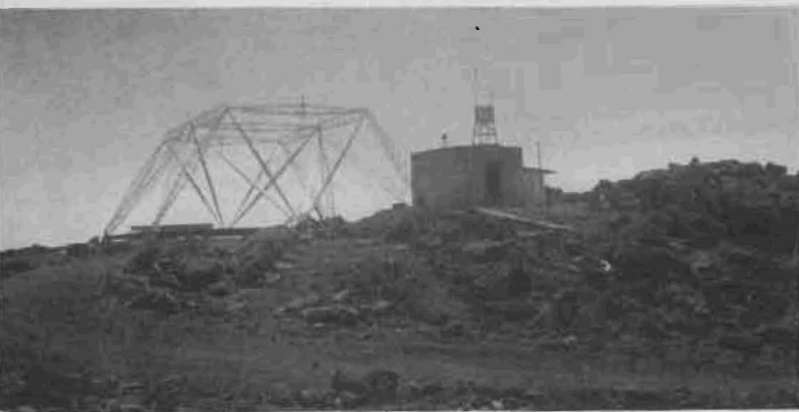
Directional antenna system on summit (10 025 feet) of Mt. Haleakala, Island of Maui. Building at right of antenna houses receivers and other equipment. Antenna system can be rotated about vertical axis passing through center of structure. Antenna forms receiving unit of a Lloyd's mirror arrangement, using reflecting surface of the ocean below, and permitting good resolution for radioastronomy studies of radiation received from stars and other sources in the galaxy. Built by Grote Reber, with cooperation of Hawaiian Telephone Co. and University.
