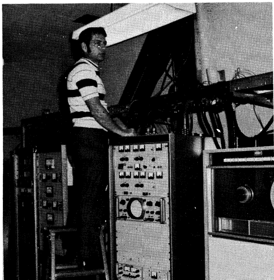
Electronics Division's Tom Dunbrack connecting control rack cables.
