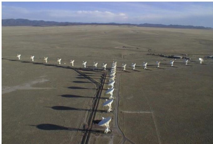
Fig. 1. Looking south, the 27 dishes of the VLA cast long, evening shadows across the Plains of San Agustin in southern New Mexico. In this configuration each arm extends ~2000 ft (600 m). Photo: NRAO/AUI/NSF/Dave Finley.
