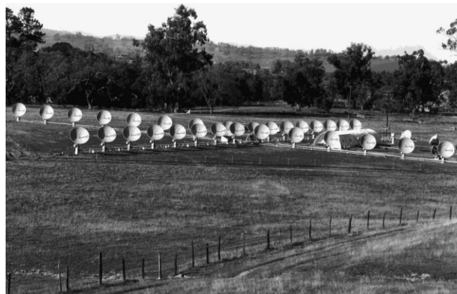
Fig. 4. Bracewell's 32-dish spectroheliograph array seen from the Southwest, observing the sun in the 1960s from his Heliopolis site near the Stanford University campus. Each cross arm is 400 ft (122 m) long. Photo: Bracewell Archives, NRAO.
