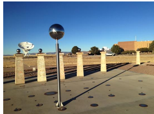
Fig. 34. A long shadow cast by the gnomon on the winter solstice of 2013 almost reaches the base of the 4h pier; the front edge of each hour-pier was placed 20 inch (51 cm) beyond the center of the winter solstice shadow (see Figs. 19 and 29). Photo: Goss.
