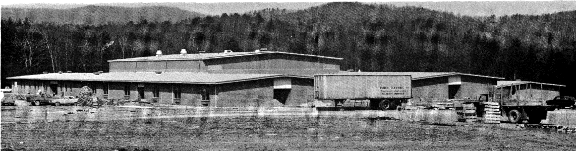
Front View of Main Building - Vocational Building Rear Right
