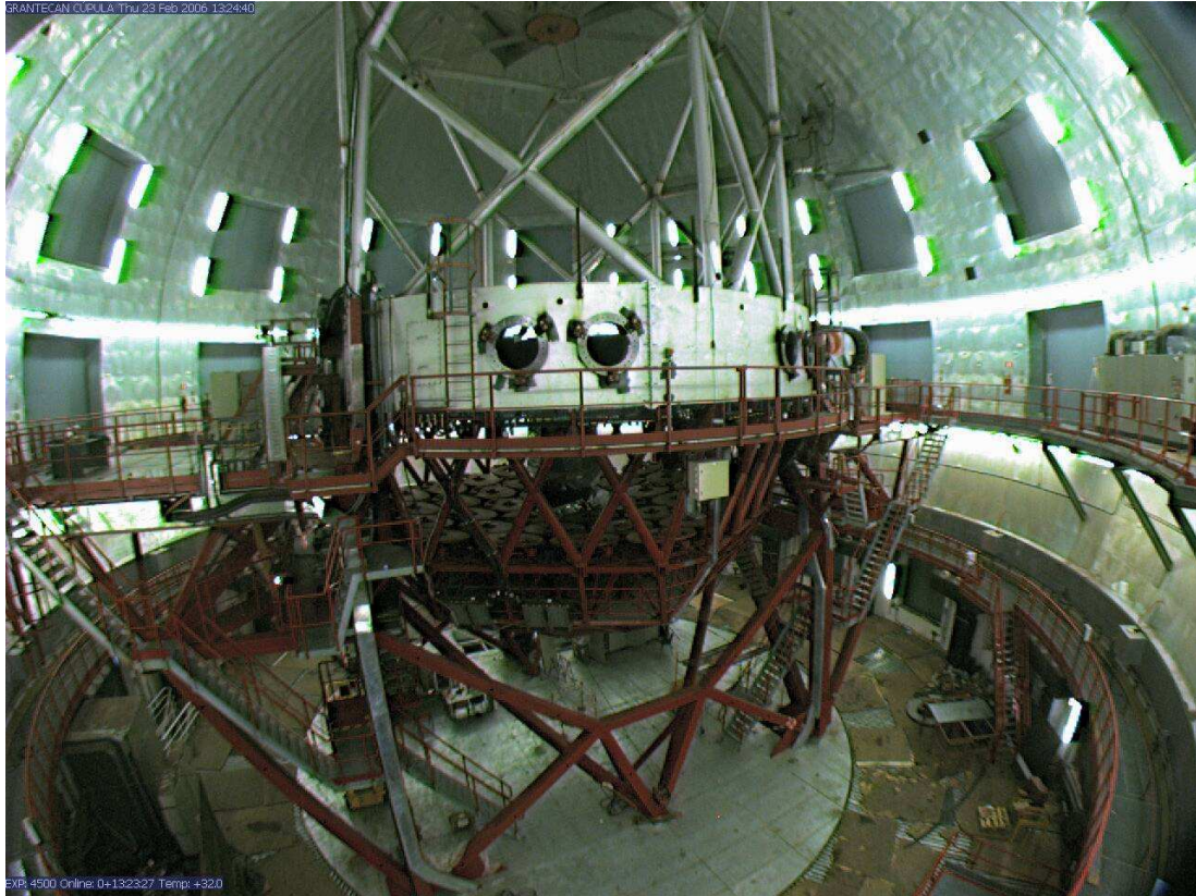
Figure 33: The GTC on La Palma during construction.
