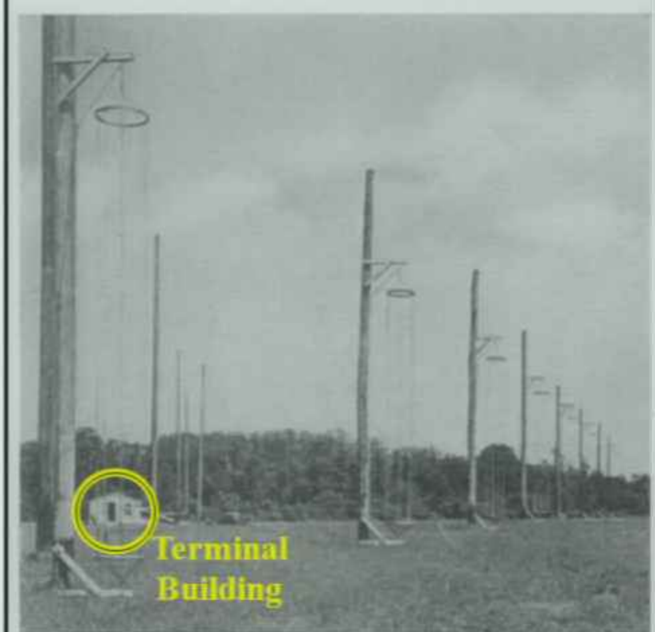
Fig. 3—The cage antennas comprising the wide-range broadside MUSA. The end cages are used as dummies.
