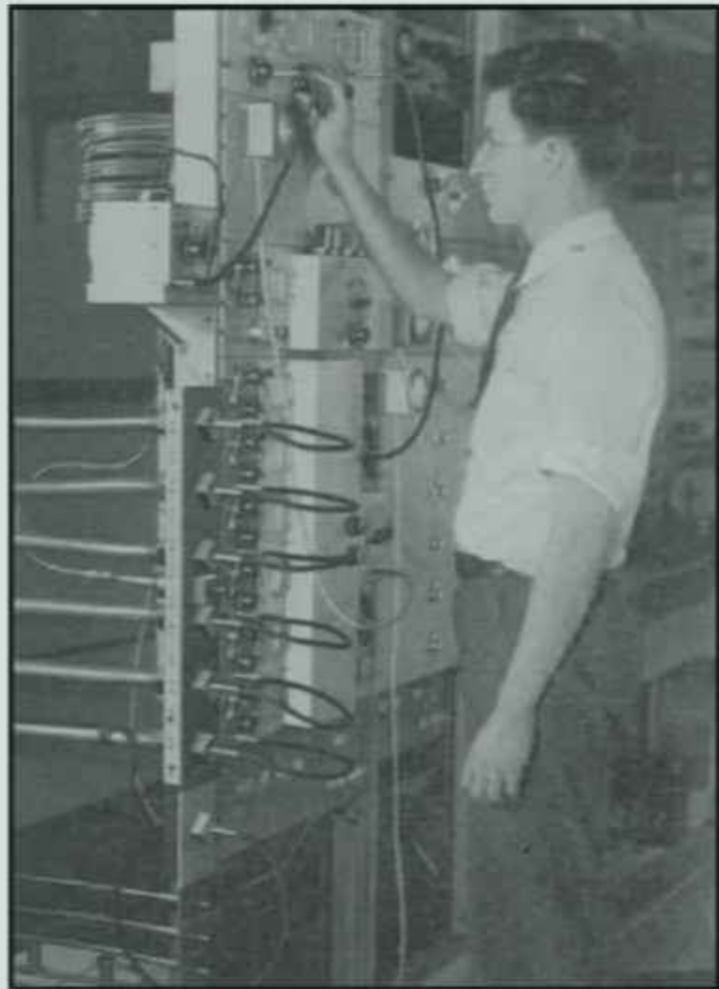
Fig. 17—View showing the six transmission lines and coaxial patch cords. The beating oscillator is mounted upon the shell and is connected to the power amplifier (which is being adjusted by Mr. Edwards) at the top of the bay.
