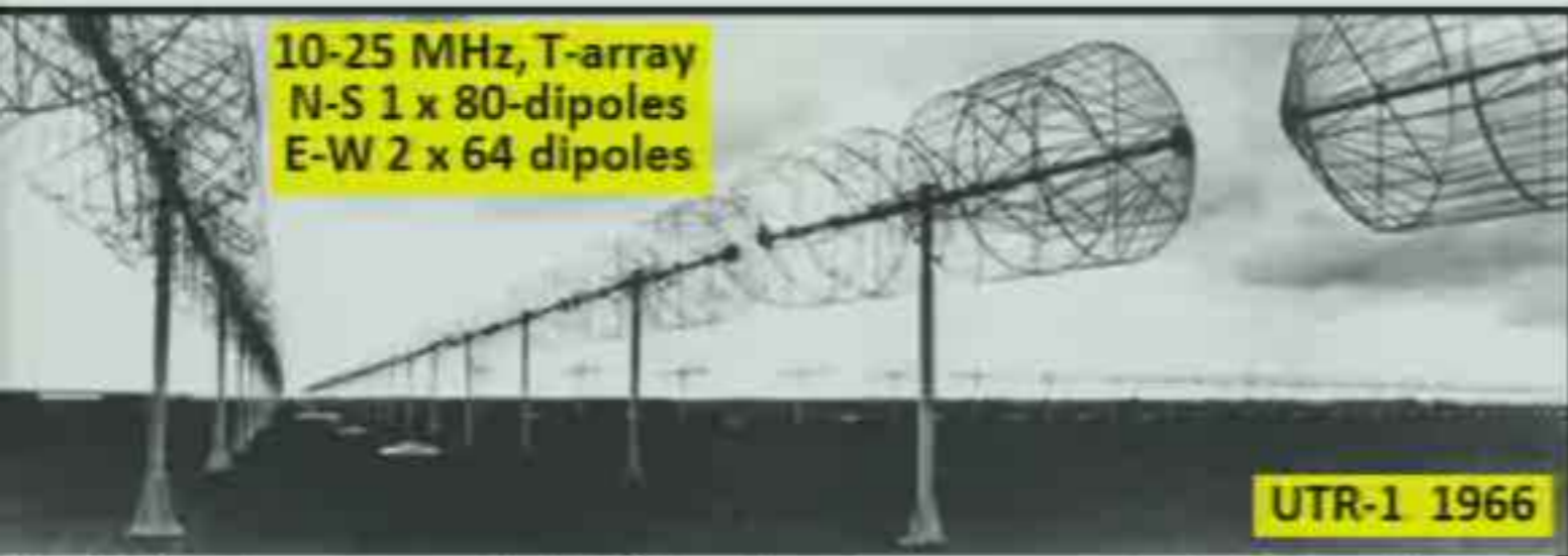
North-South antenna of the UTR-1 radio telescope, comprised of 80 oscillators
