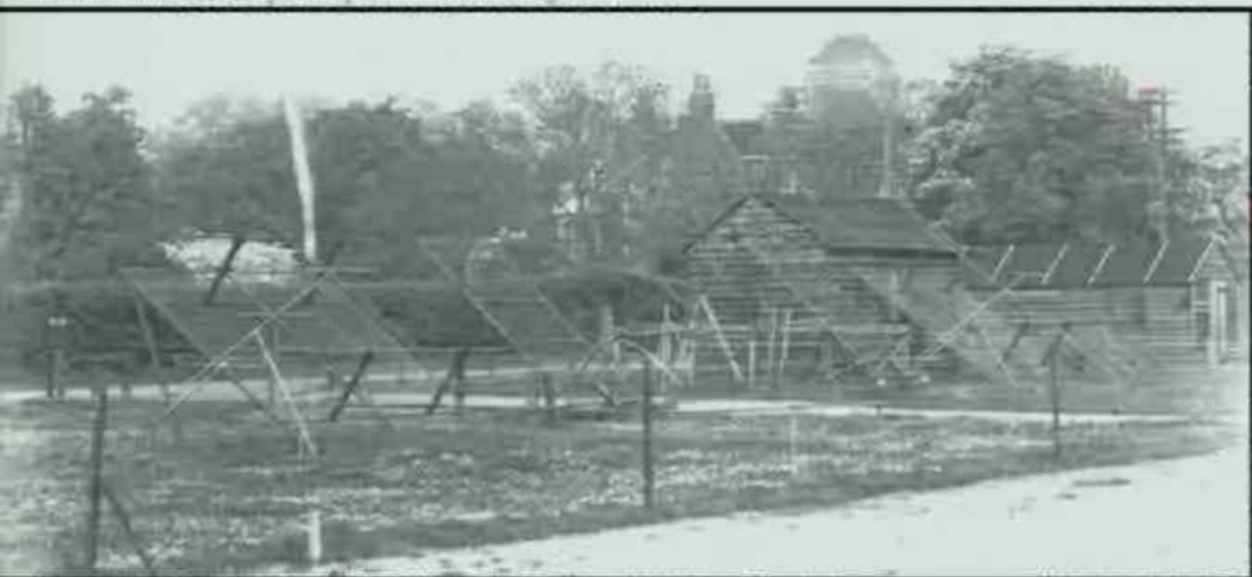
Figure 8.2. First observing hut (leftmost) and early antennas of Ryle's group, circa 1948 at the "Rifle Range" field station off Grange Road, Cambridge (see Fig. 8.3). Several solar interferometers are shown. From the left, (1) (in front) 80 MHz Yagi; (2) (behind) 80 MHz 4-dipole broadside array with reflecting screen; (3) 175 MHz 8-dipole array; path; (4) antenna paired with 3; (5) (in front) pair with 1; (6) (behind, cubical structure higher than shack) 214 MHz 4-Yagi array (operated as a single antenna, based on a wartime "Lightweight Warning" set); (7) pair with 2; (8) alternate pair with 3 (with polarization crossed). Ryle's house is off to the left and the tower of the main University Library is visible in the background.
