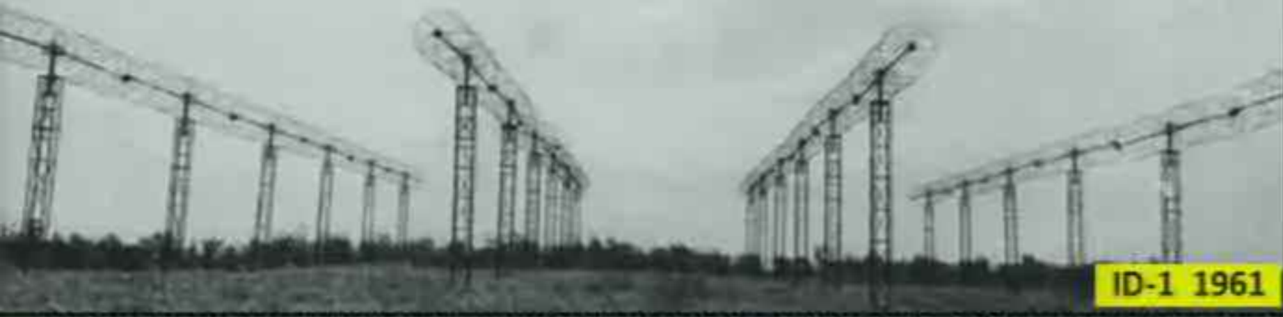
Antenna arrays of the second version of the ID-1 interferometer
