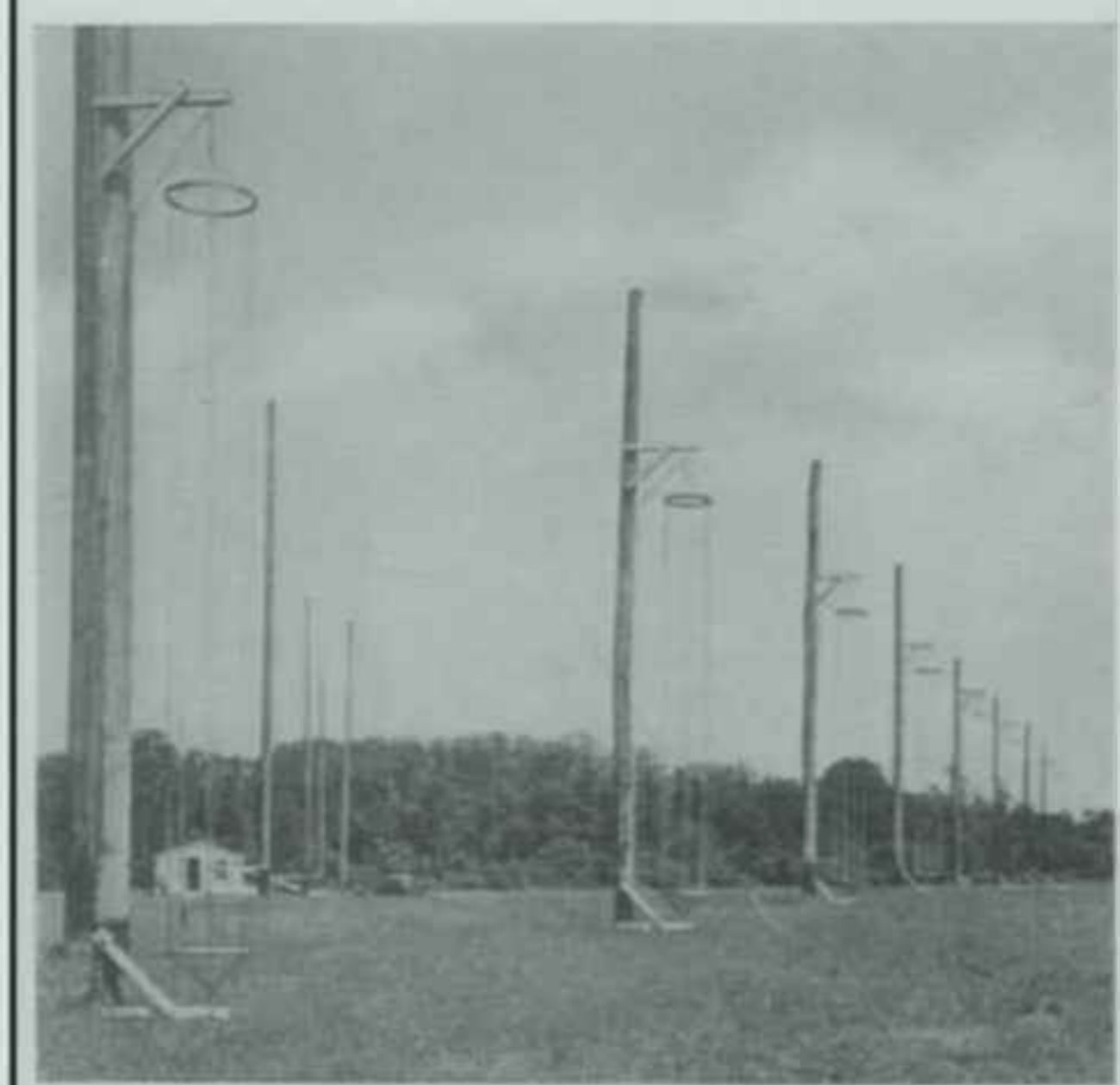
Fig. 3—The cage antennas comprising the wide-range broadside MUSA. The end cages are used as dummies.
