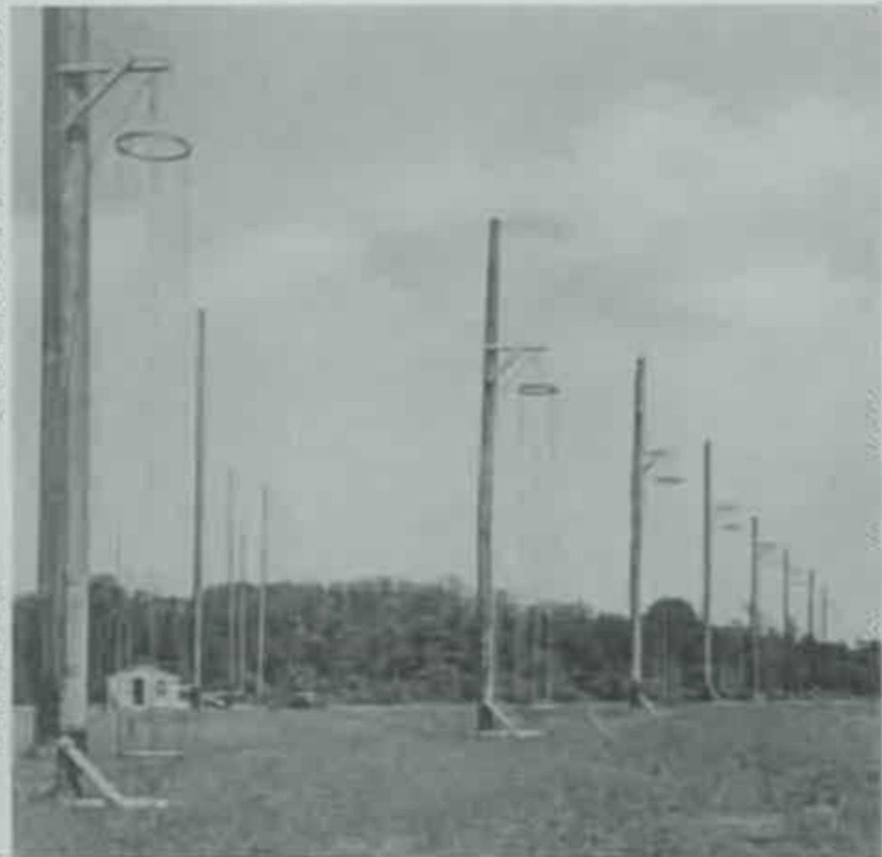
Fig. 3—The cage antennas comprising the wide-range broadside MUSA. The end cages are used as dummies.
