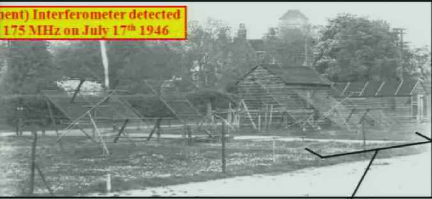
Figure 8.2. First observing hut (leftmost) and early antennas of Ryle's group, circa 1948 at the "Rifle Range" field station off Grange Road, Cambridge (see Fig. 8.3). Several solar interferometers are shown. From the left, (1) (in front) 80 MHz Yagi; (2) (behind) 80 MHz 4-dipole broadside array with reflecting screen; (3) 175 MHz 8-dipole array; path; (4) antenna paired with 3; (5) (in front) pair with 1; (6) (behind, cubical structure higher than shack) 214 MHz 4-Yagi array (operated as a single antenna, based on a wartime "Lightweight Warning" set); (7) pair with 2; (8) alternate pair with 3 (with polarization crossed). Ryle's house is off to the left and the tower of the main University Library is visible in the background.
