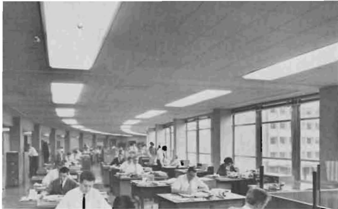
A facelift for the interior lighting of Qantas House in Sydney was given by installing fittings made from 'Perspex' Diamond 030 acrylic sheet. Over 1,000 fittings were installed, mostly in the 4' x 2' size.
