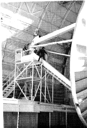
Later (or was it earlier), Rick Howard and others installed the rotating subreflector at the prime-focus. Rick appears to be contemplating a fast downward slide. He didn't.
