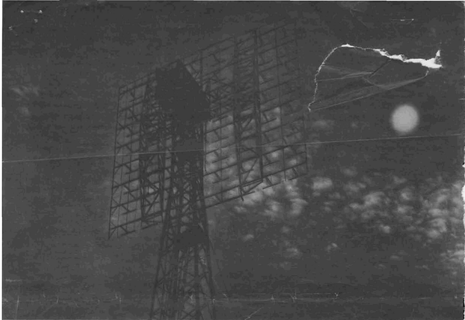
The "bedspring" antenna at Belmar, New Jersey.
