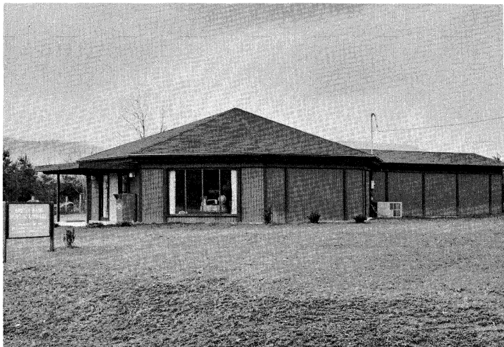
Library and activity room addition.
