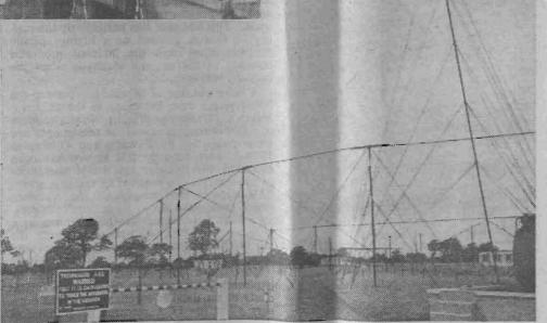
A recent photograph showing part of the 220st, aperture fixed radio telescope which has a paraboloidal surface formed by a series of wires supported around the perimeter by posts 24st, high. The aerial at the focus is carried on a 120st, mast, which is tilted to displace the beam from the zenith. Above: Recording apparatus used with the telscope; the chart shows that the radio star in Cygnus has just passed through the beam of the aerial system.
