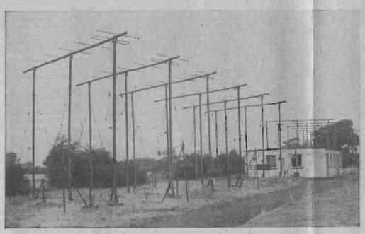
The aerial system used for the continuous survey of meteors by the radio echo technique. In the small building is the apparatus which has now been working for several years and has provided information about meteoric activity uninterrupted by cloud or daylight.
