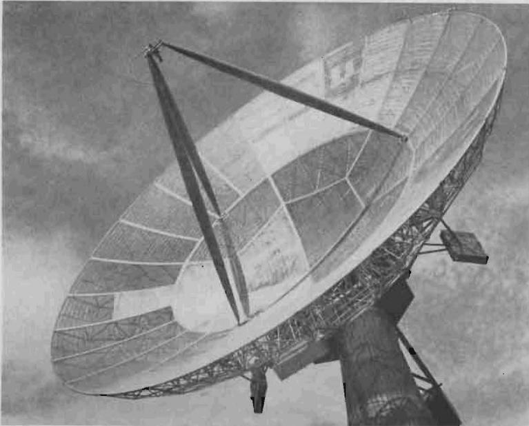
FIG. 2. The 60-foot George R. Agassiz Radio Telescope. Photo by Robert E. Cox with kind permission of Sky and Telescope.
