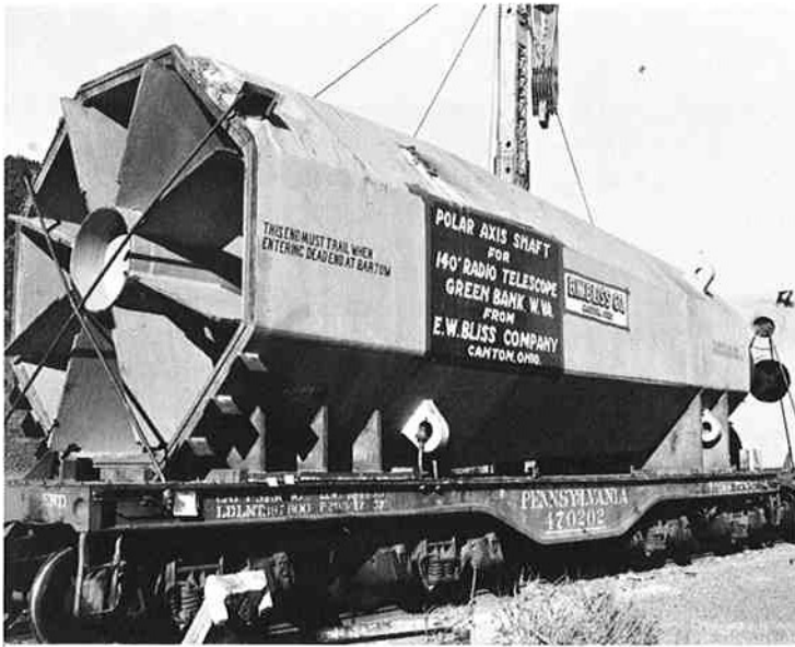
FIGURE 21. Two sections of the polar shaft that were the first sub-assemblies of the telescope shipped to Green Bank. The larger section weighs 160 tons.
