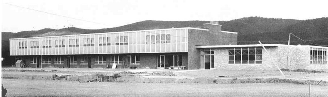
FIGURE 25. The Residence Hall, with cafeteria attached at the south end. The sixteen rooms on the second floor are served by a lounge and entrance hall next to the cafeteria. The four first-floor apartments have individual entrances sheltered by the overhang of the rooms above.
