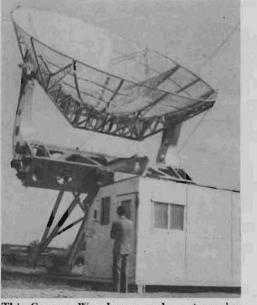
This German Wurzburger radar antenna has been adapted for use with Reber's equipment for receiving solar radiations and set up at Sterling, Va. Housing is German prefab steel shack.
