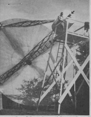
Grote Reber is shown with his great "mirror." He is atop a 20-foot scaffold adjusting the receiving equipment (arrow) for 160-megacycle tests, the first frequency he used successfully.
