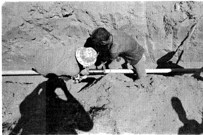
If all goes well, i.e., no sand in the threads, this is how two 16-ft. sections of waveguide are coupled together.
