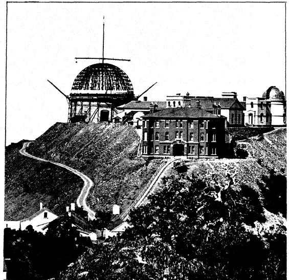
The dome of the 36-inch reflector was the last unit of the main Observatory building to be completed. The 3-story brick building in the foreground was a dormitory which was severely damaged and replaced after an earthquake in 1911. The photograph was taken in 1887.
