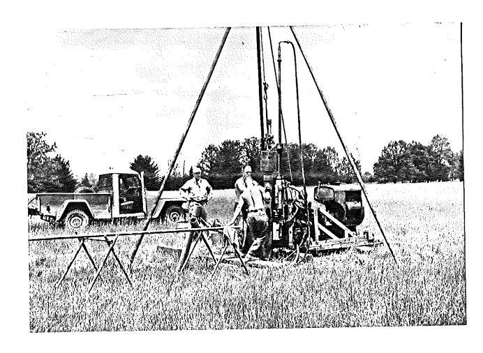
Photograph Showing Drilling of Core Test Hole Near Green Bank, W. Va.
