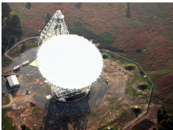
Figures 1 & 2. Views of the Green Bank Telescope from above and below; the primary mirror is 100 m across.
