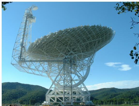
Figures 1 & 2. Views of the Green Bank Telescope from above and below; the primary mirror is 100 m across.
