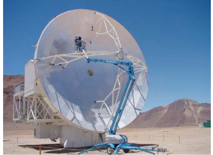
Fig. 1. APEX 12 m antenna located on the Llano Chajnantor at 5100 m altitude in Northern Chile. On the picture, a crew of two people is adjusting the 5-screw panels to improve the surface accuracy. This is normally performed once a year after a holography session and is needed to allow efficient THz observations.
