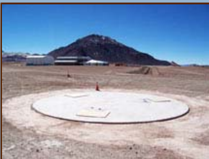
Figure 1. Antenna station A93. The AOS Technical Building is between A93 and Chajnantor, and the Transporter Hangar is at left. (Photo S. Cabezon)
