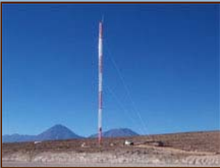
Figure 4. A new holography system, built at the NRAO Technology Center, will be assembled at the OSF Technical Building. The transmitter will be mounted atop the recently finished holography tower. The Licancabur volcano (left) and Juriques (right) are in the background.
