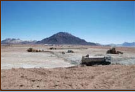
Figure 2. Grading proceeds at the center of the array. Antenna station A93, the Technical Building, and the Hangar are in the distant background against Chajnantor.
