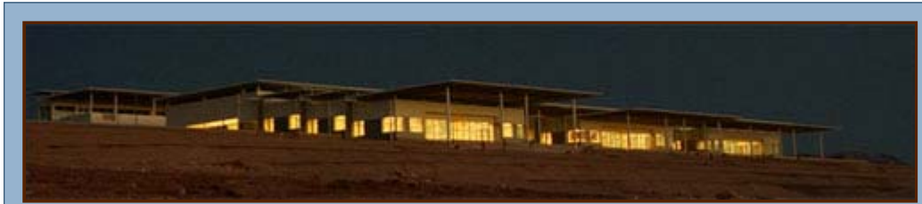
Figure 2. Work continues past sunset in the new OSF Technical Building, seen here just before drawing of the nightshades
